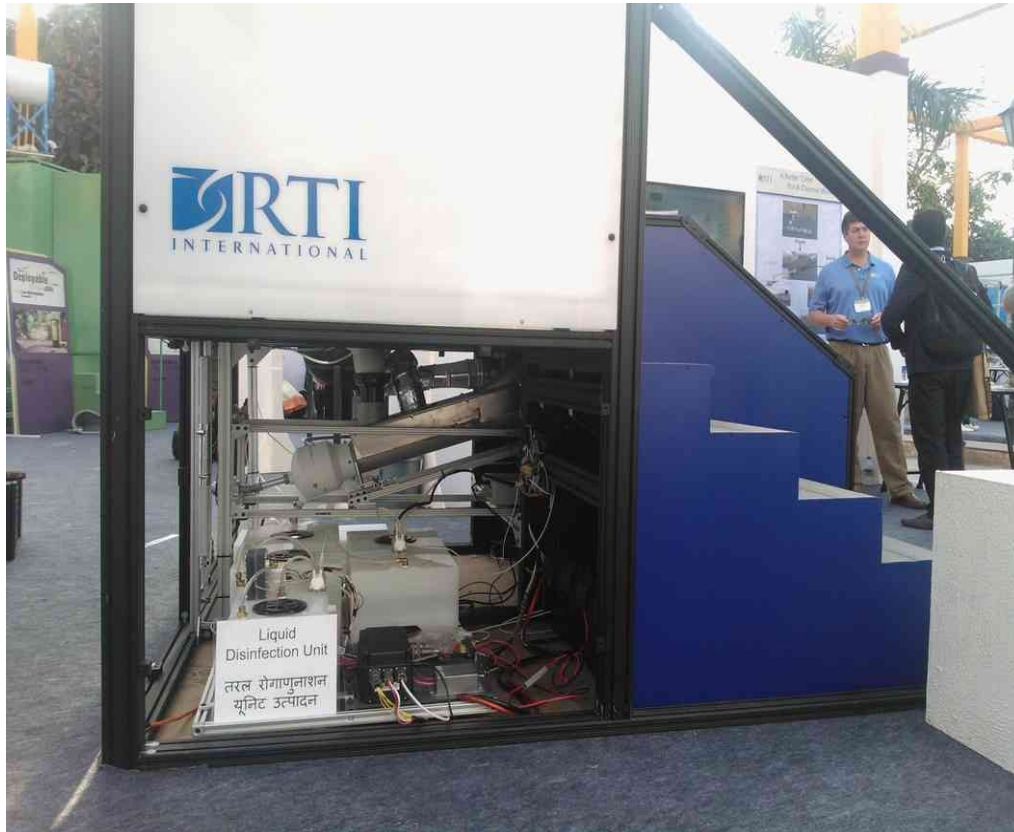
Liquid treatment components contained under the toilet platform, CC-BY-2.0 SusanASecretariat
